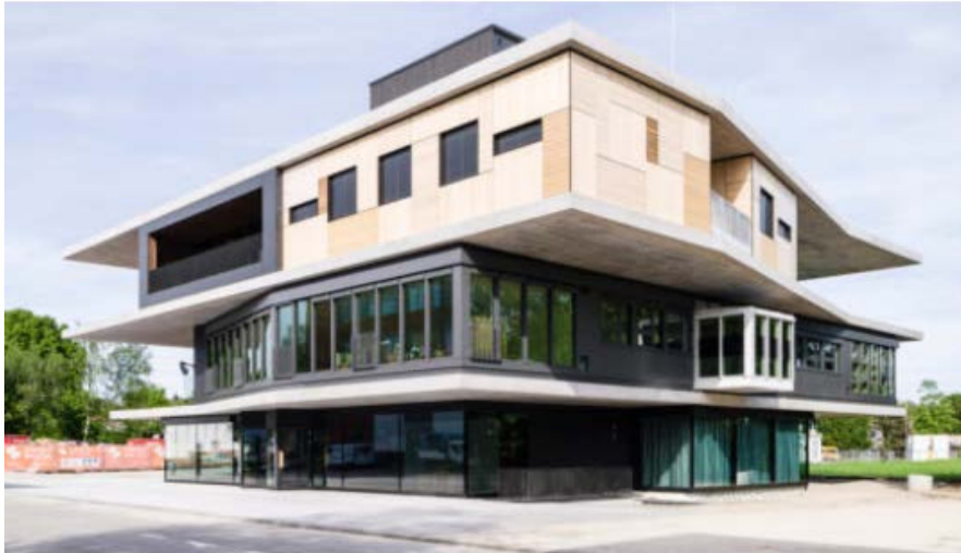
Fig. 5 The DFAB House in Switzerland: shows the 3d printing concrete application (DFAB HOUSE 2018).
